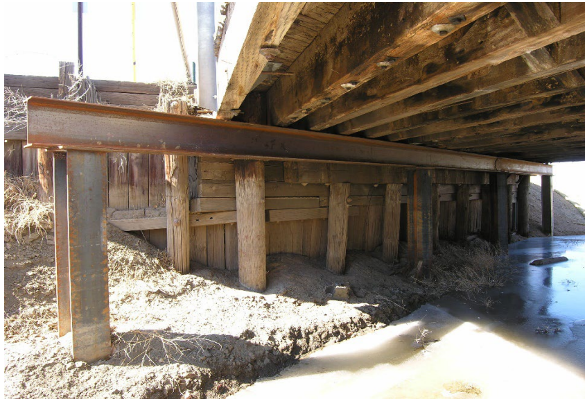
Fig. 16.12(H)-7 Photo of New Support Bent near Abutment
