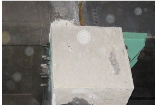
Fig. 16.12(F)-4 Photo of Corbel Placement and Pier Cap repair
