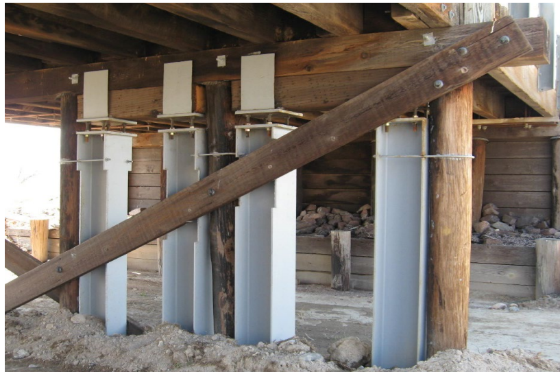
Fig. 16.12(G)-6 Photo of Adding Columns to a Pile
