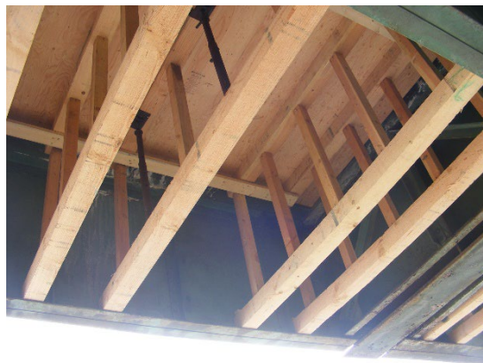
Fig. 16.12(I)-2 Photo of Deck Falsework
